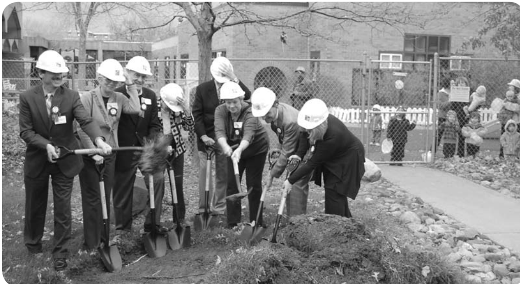
Tots from FUNDamentals look on with excitement during the groundbreaking for the new addition.
