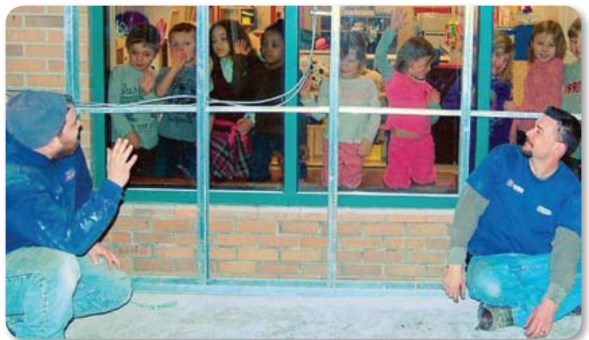
Children gaze out in astonishment at the progress of their new FUNdamentals building addition, as two construction workers, Zach Taylor and Chris Wurgler smile and wave back.
